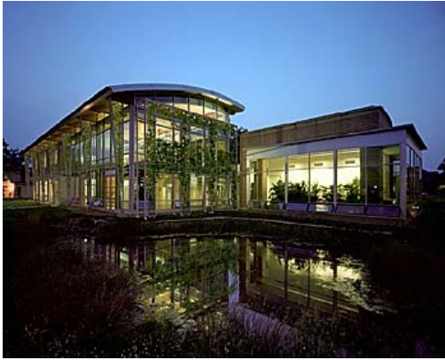
Figure II.5. South facing windows at Oberlin College's Lewis Center for Environmental Studies.
